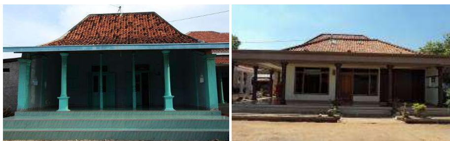
Figure 8: Columns used in traditional (left) and present-day architecture (right).
