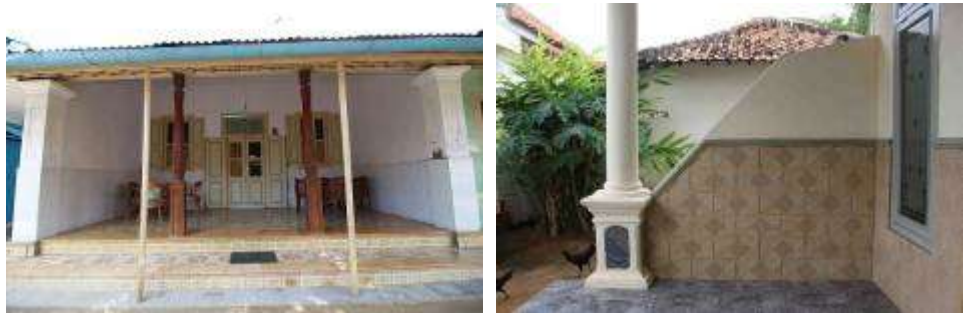
Figure 7: A full wall (left) and a half wall on the side of the porch (right).
